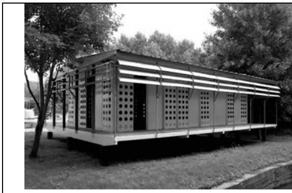
Figure 3.18 Exterior view of the Tropical House
