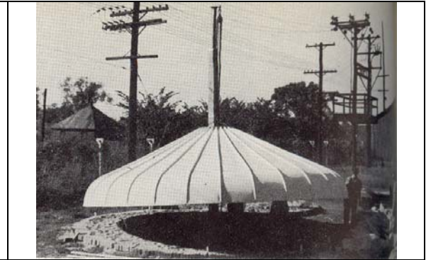
Figure 3.13 Mast supporting DDU structure
